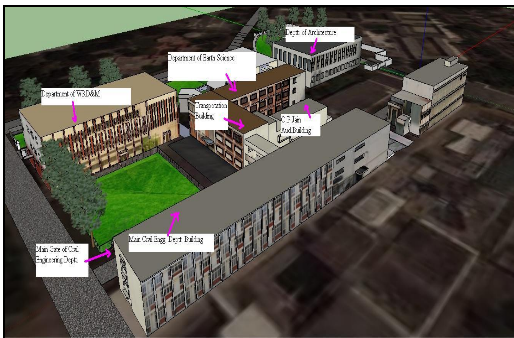
Figure 4: Another View of 3D model of Department of Civil Engineering, IIT-Roorkee, India
