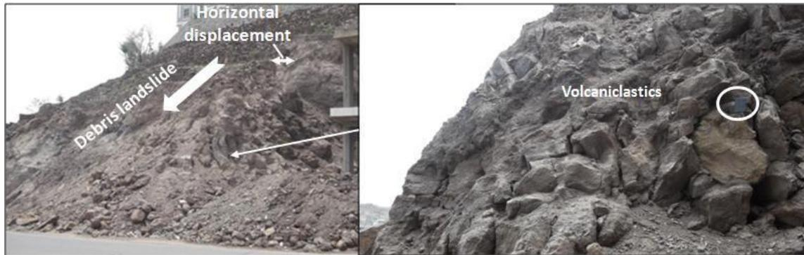
**Figure 33:** Field photographs showing the debris landslide in intensely weathered basic volcaniclastics-Tb2 located in the southeast NWRA, Ussayfra area. Note the horizontal displacement (about 1.4m) and the movement direction (EW) of landslide. Field notebook height 20 cm (inside white circle)
