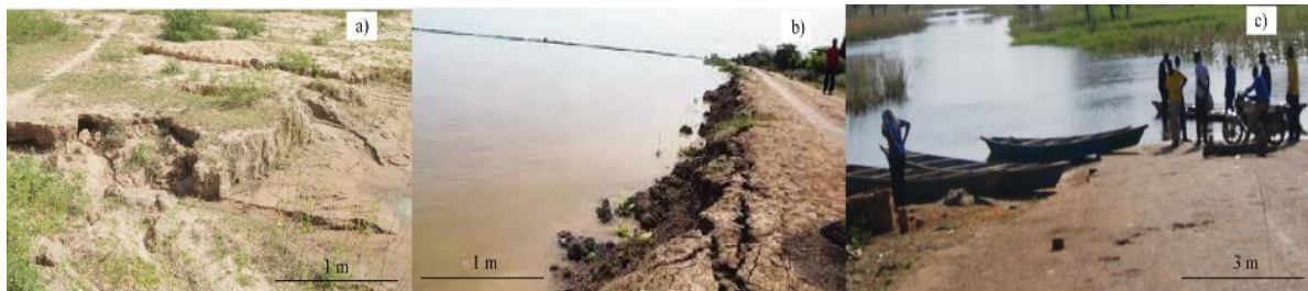
Figure 20: Soil erosion at Yagoua (a), banks of Logone River (b, c))
