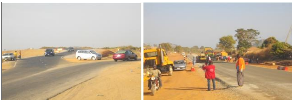
Plate 1: Road Construction Connecting Kuje to Gwagwalada at Pasali Area
