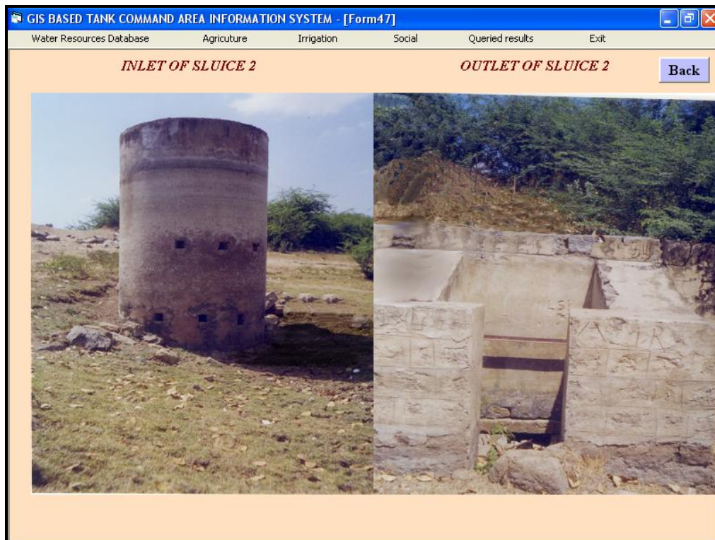
Figure 6: Menu Shows the Condition of Inlet and Outlet of Sluice 2
