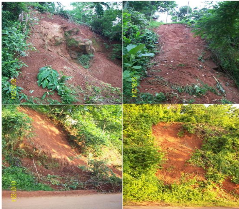
Figure 2: Few landslide sites in the field
